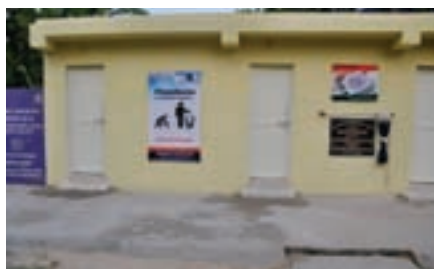
Toilets constructed by Kolkata North Commissionerate in Parivar School, Picnic Garden Road, Kolkata
