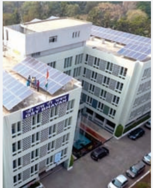
Aerial View: Solar Power Plant at GST Bhavan, Pune.
