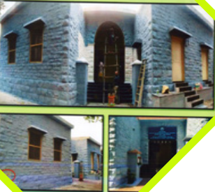
OFFICE BUILDING WAS REPAINTED
