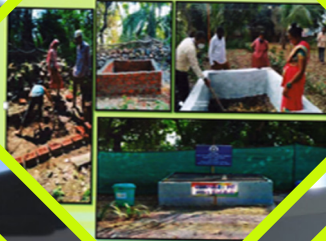
CONSTRUCTION OF COMPOST PIT
